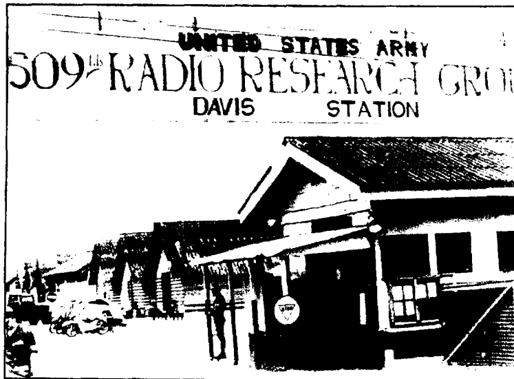
(U) Entrance to Davis Station
