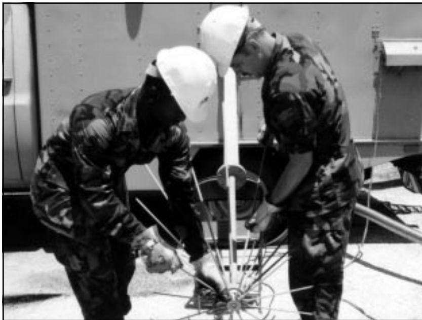
These airmen set a communications antenna.
