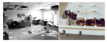
Figure A-11. Images of blast damage at Henderson, NV, courtesy of the City of Henderson, NV, similar to that expected at the outer edge of the LDZ.
