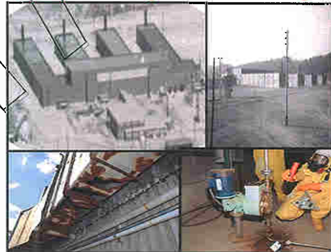
Deteriorating Duct Work
