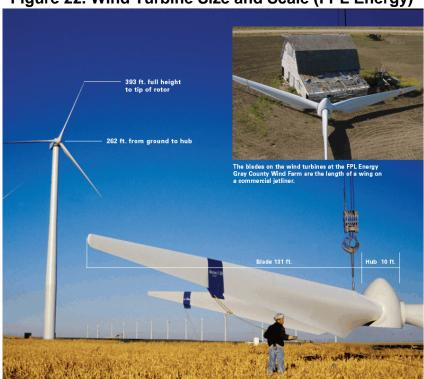
Figure 22. Wind Turbine Size and Scale (FPL Energy)
