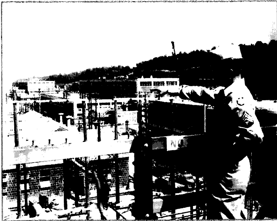
The Y-12 Plant was established in 1943 as part of the Manhattan Project with a mission to separate uranium-235 from natural uranium using the electromagnetic separation process. Pictured is a view of the Y-12 Plant looking east in 1944.
