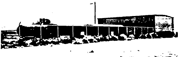
Fig. 3. Present filter test facility, showing tanks and building housing wind tunnel.
