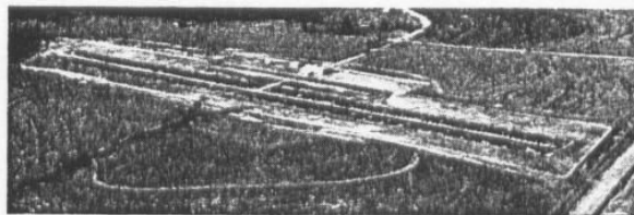
Fig. 9—The Jordan Lake transmitting site.
