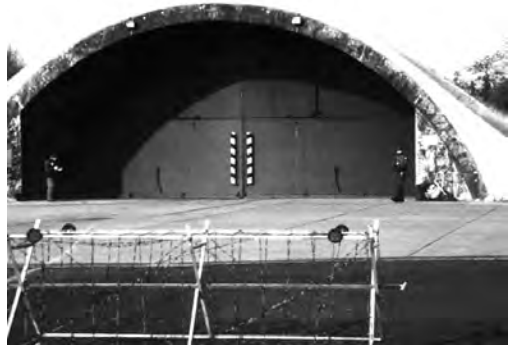
Figure 4.8 Munitions Storage Igloo
